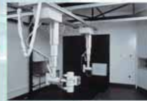
General View of the X-ray room for Large Animals
